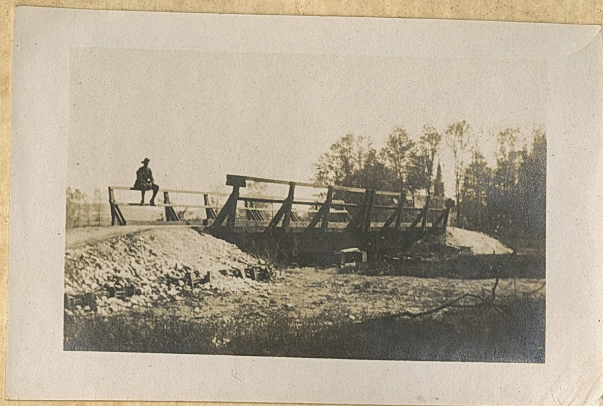
A Military Bridge between Querrieu and Pont Noyelles
