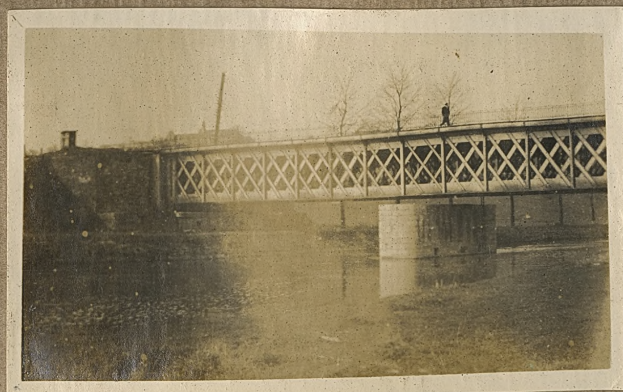
The railway-bridge over the river
