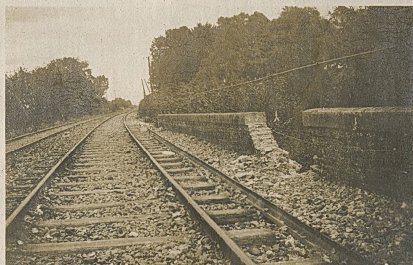
The Bridge from above
