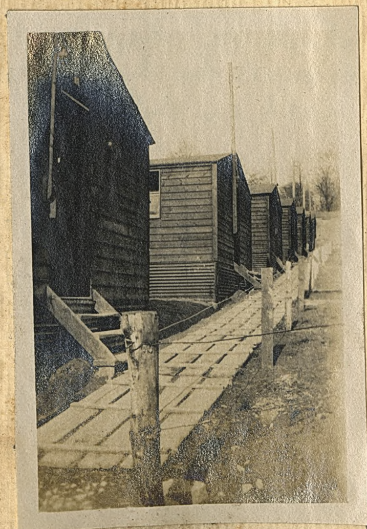
Huts of Signal Section
