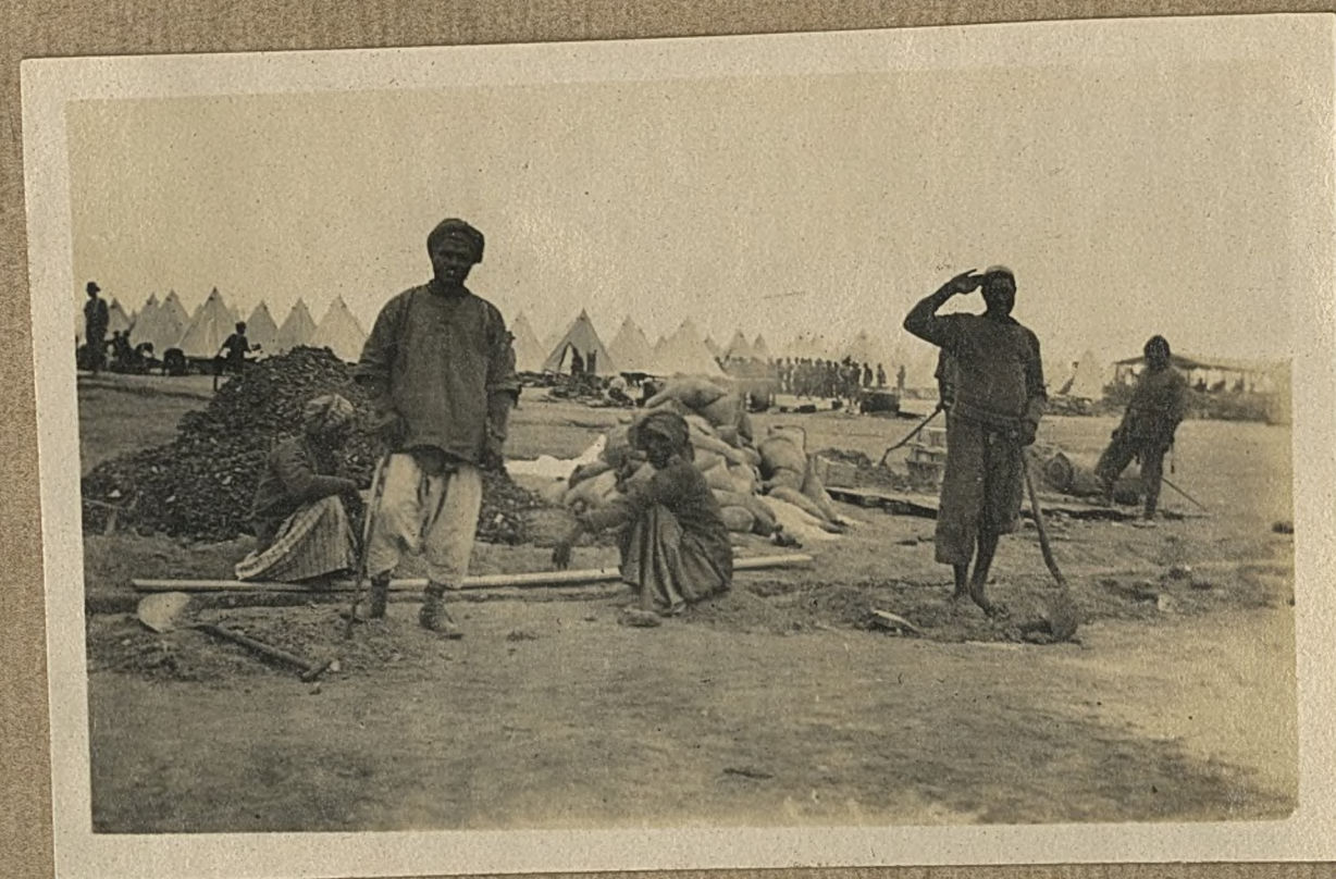
Making a drain
