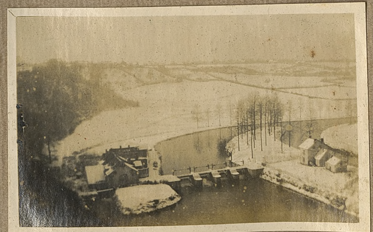
The flood-gates at Thuin - winter
