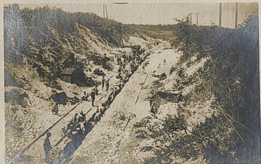
Digging the Cable-Trench
