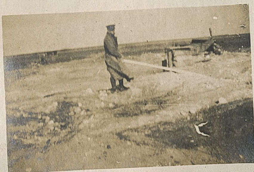
Burred Cable - Laying out the guiding rope
