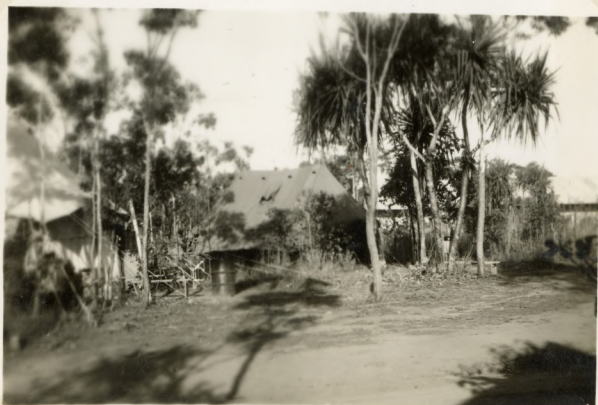
Adelaide River North Side
