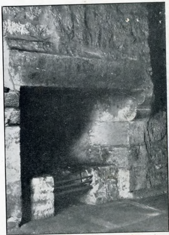
PROVAND'S LORDSHIP Fireplace in South Mid-Chamber
