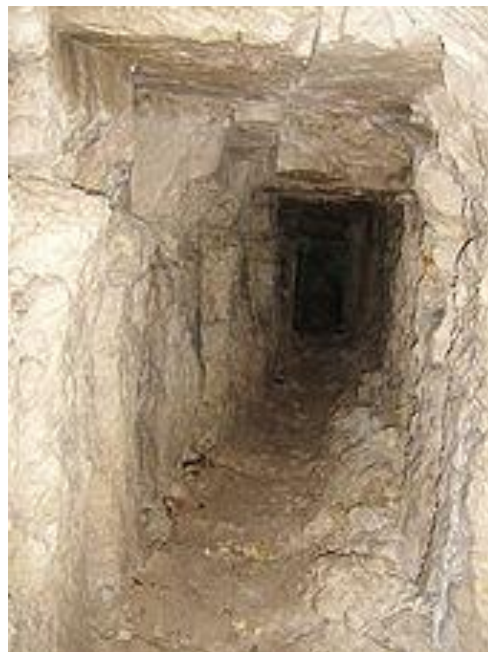
Fighting tunnel in Vimy sector
