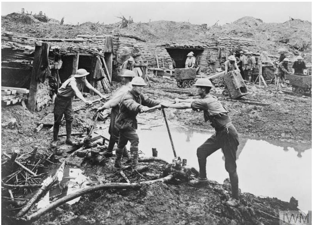
Tunnellers pumping water out of trenches and tunnels
