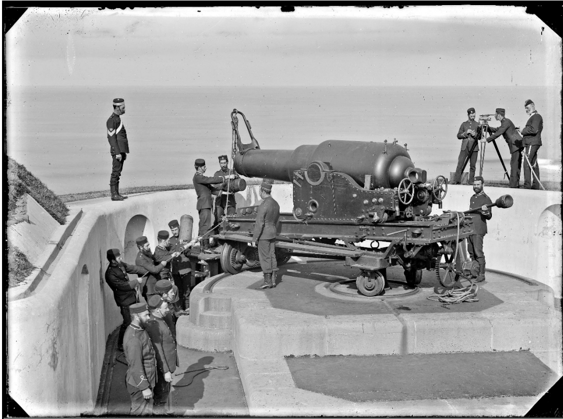
Figure 3. Artillerymen loading a 9inch RML gun at Fort Scratchley (1882-1891) Note the artillerymen using what looks like a surveying instrument to obtain range and baring to the target. It is also clear that loading the gun was quite an effort. (Snowball Collection, University of Newcastle)
