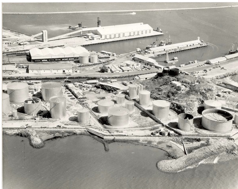
Figure 5. Aerial photograph of harbour installations showing reclamation works and expansion of oil storage facilities, 1966. (Townsville Port Authority; Lawrence, Brown, McPhee and Slaughter 2006, 69, Fig 7)
