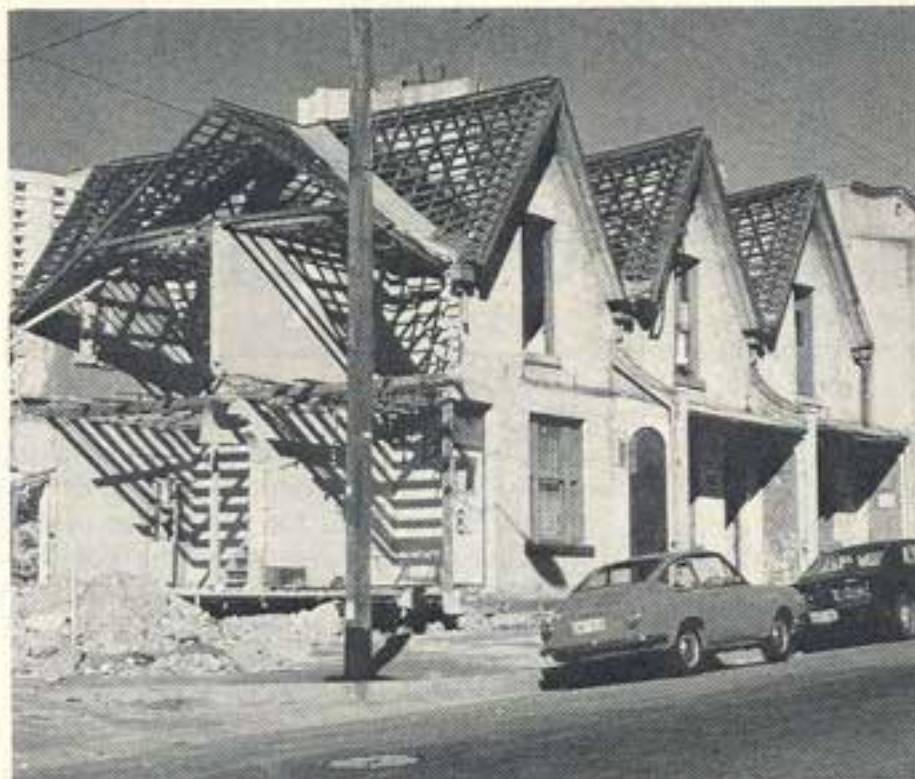
During restoration Terrace housing in Woolloomooloo, photographed by John Devenish.
