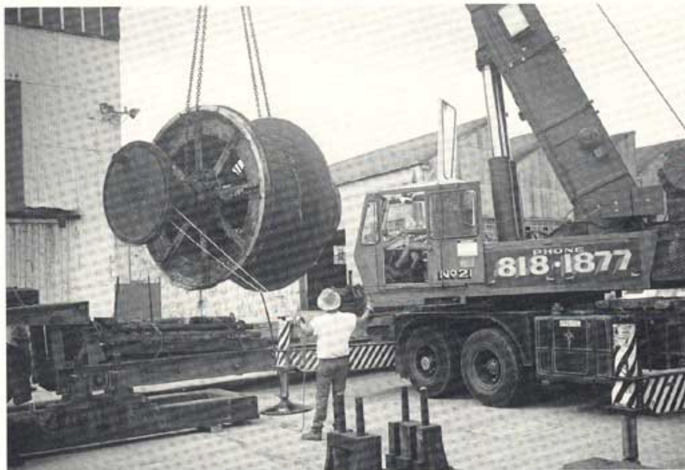
Components of the Hebburn Colliery winding engine being unloaded at the Leichhardt Workshops of the Public Works Department.
