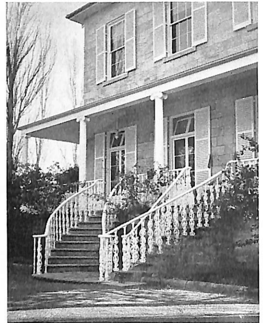
"From the high-pillared verandah on the other side of the house, two stairways curve to meet, forming a complicated and delicate design."
