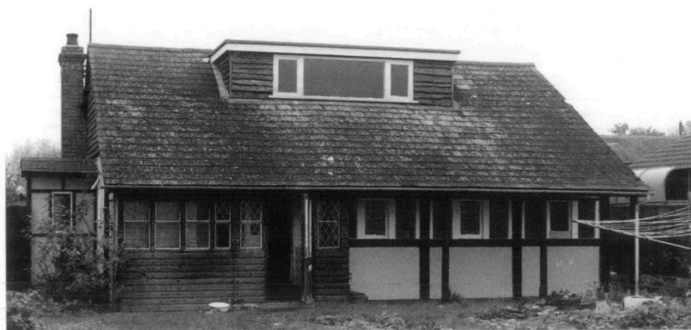
Who would have thought this house contained two antique railway coaches in original condition? The retirement home for the S&D coaches, now being demolished and yielding up its treasures. (Photo: S. Ehrlicher).
