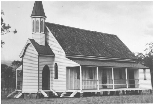
Caboonbah Undenominational church with shingle roof
