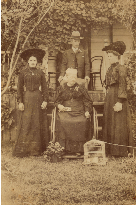
Mrs. R.D. Soden in the wheel chair that required the removable verandah rail for her direct entry to Church from a dray.
