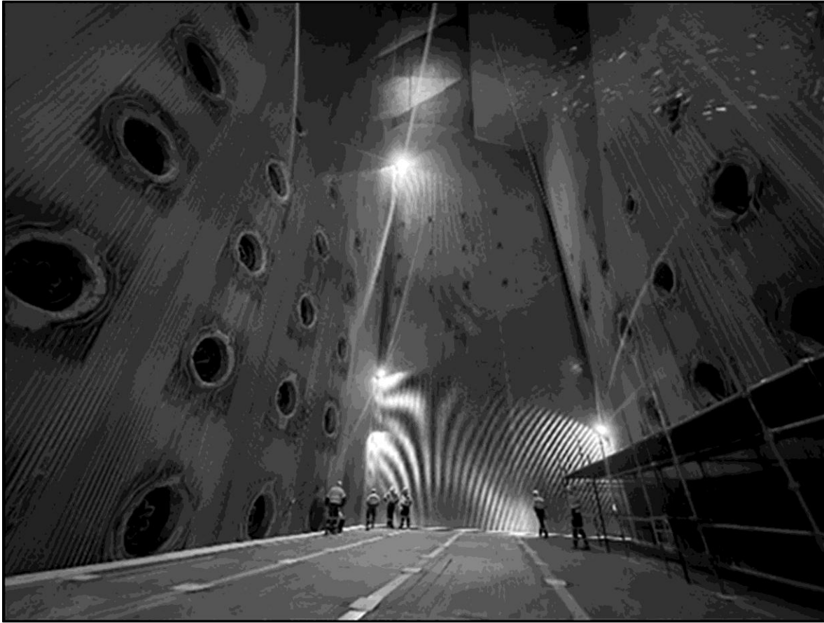
Figure 78 Boiler ‘Dance Floor’, October 2023 (Origin Energy)
