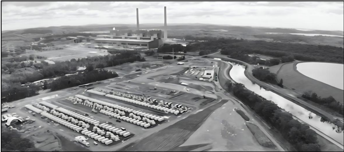
Figure 7 Eraring Battery site with the power station in the background. (Origin Energy)
