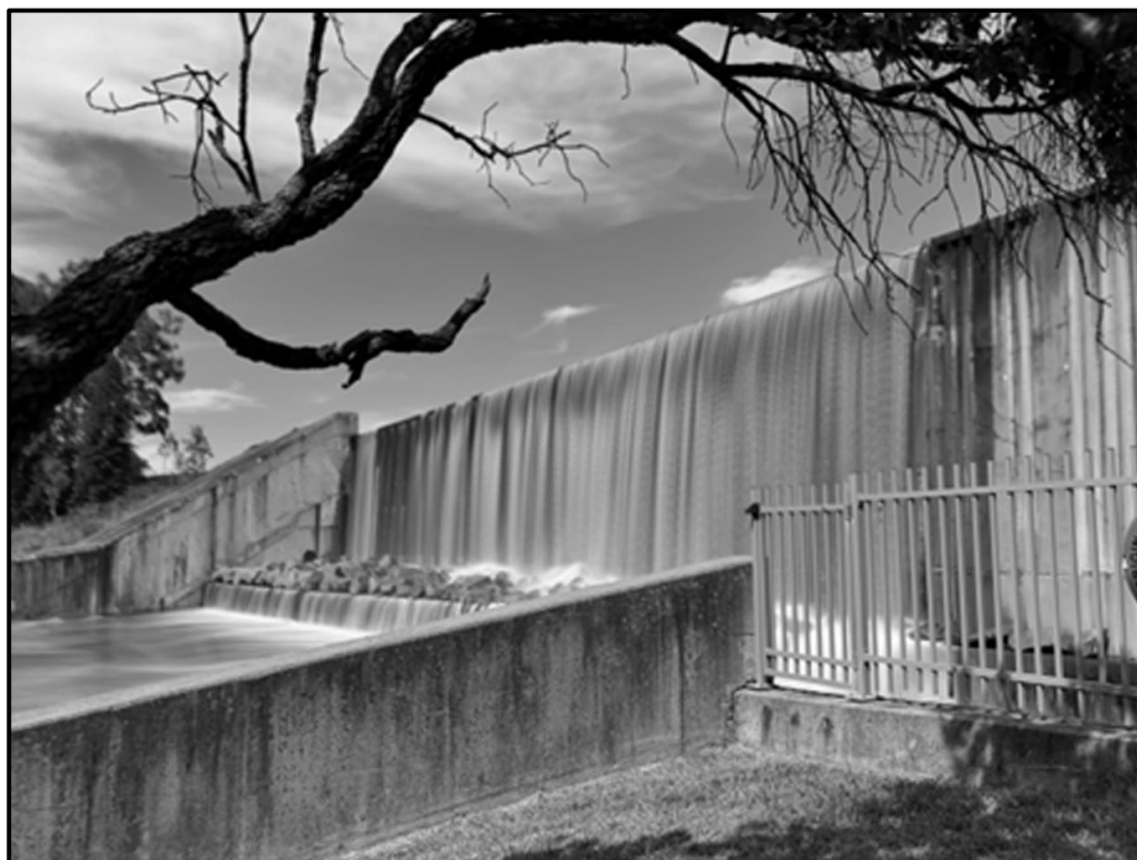
Figure 59 High-Level Canal overflowing, October 2024 (Ken Thornton)
