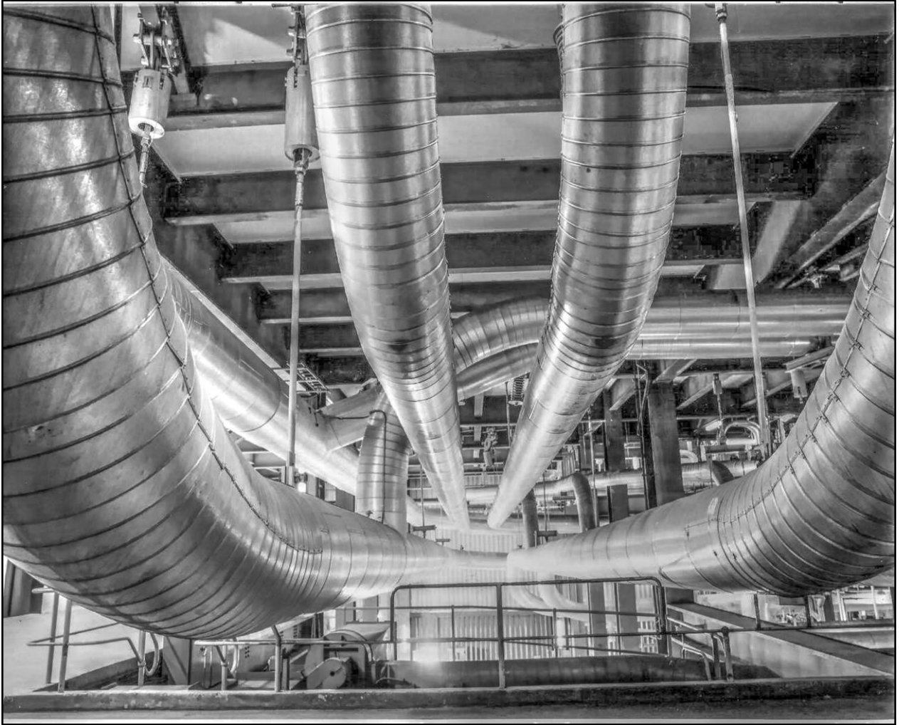
Figure 62 Steam pipes to and from boiler, 2023 (Ken Thornton ??)
