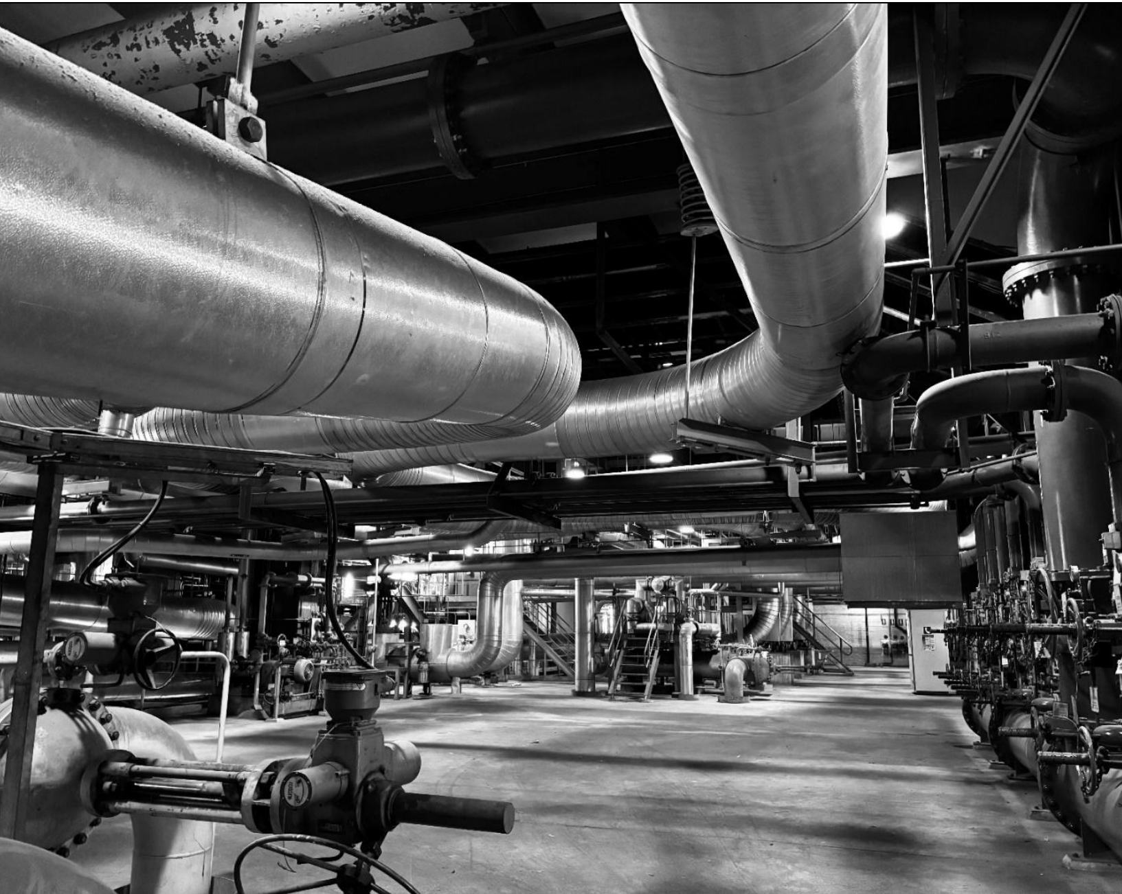
Figure 27 Mezzanine Floor November 2024 (Ken Thornton)
