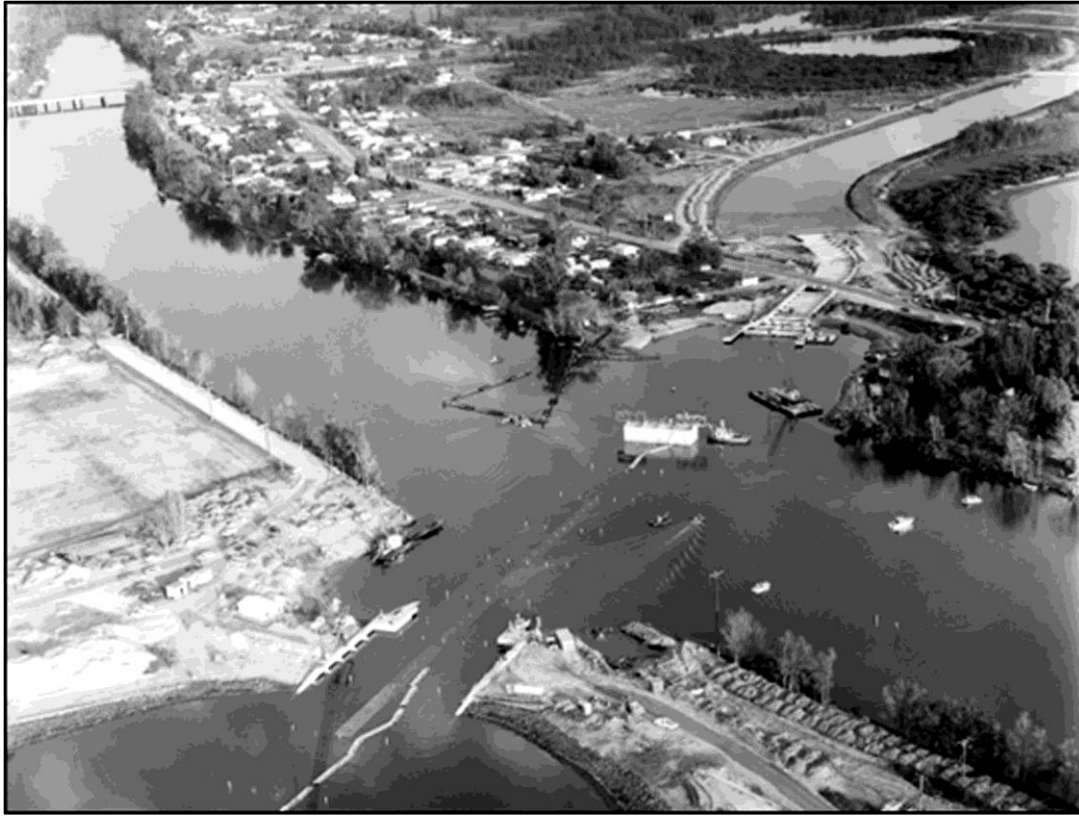
Figure 57 Cooling water caisson being floated into place before being sunk into a trench in Dora Creek, January 1980 (ECNSW)
