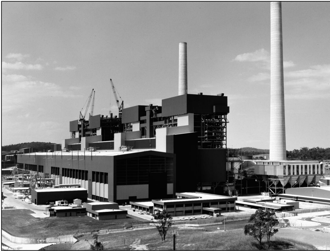
Figure 3 Units 3 & 4 under construction between November 1982 and July 1983 (ECNSW CT7.0011)
