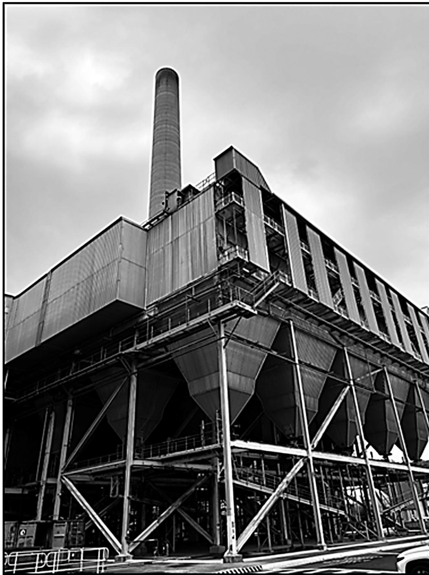
Figure 55 Fabric Filters, November 2024 (Ken Thornton)
