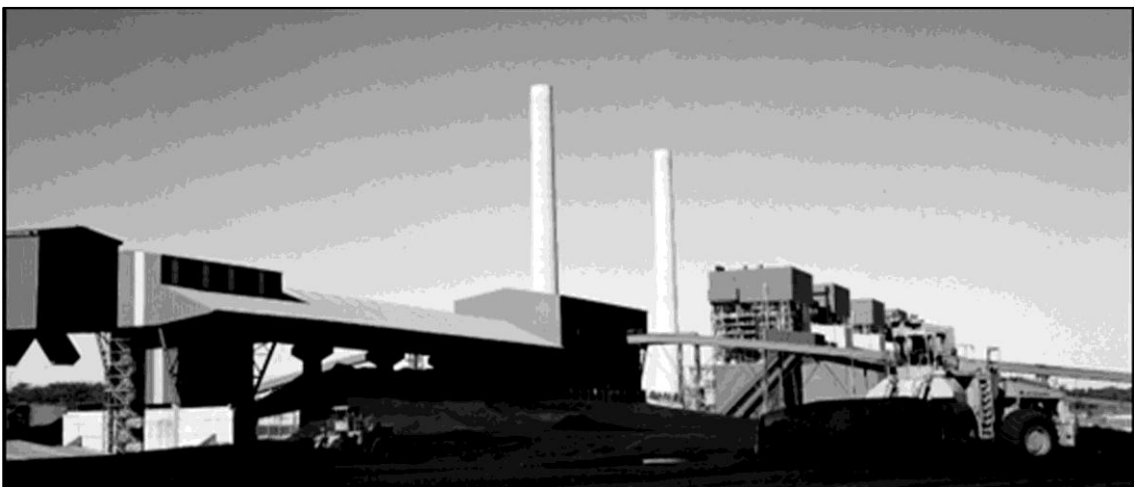
Figure 49 Coal Stack, May 1984 (ECNSW CT7,0003)
