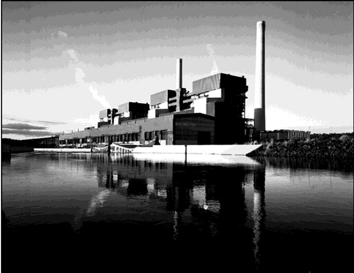
Figure 35 From the southwest, June 1984 (ECNSW 13769)
