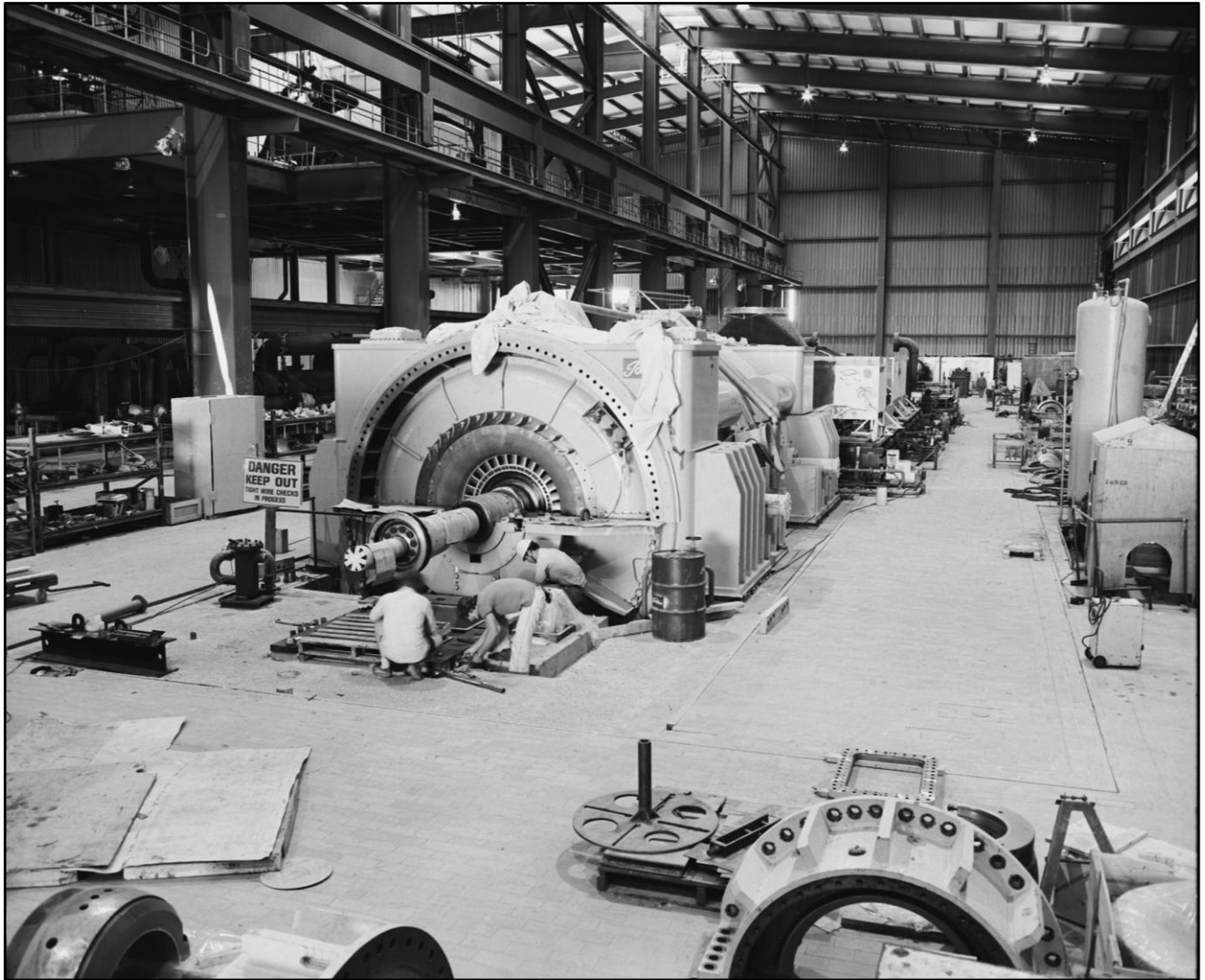
Figure 41 Turbine Floor, November 1980 (ECNSW 13328)
