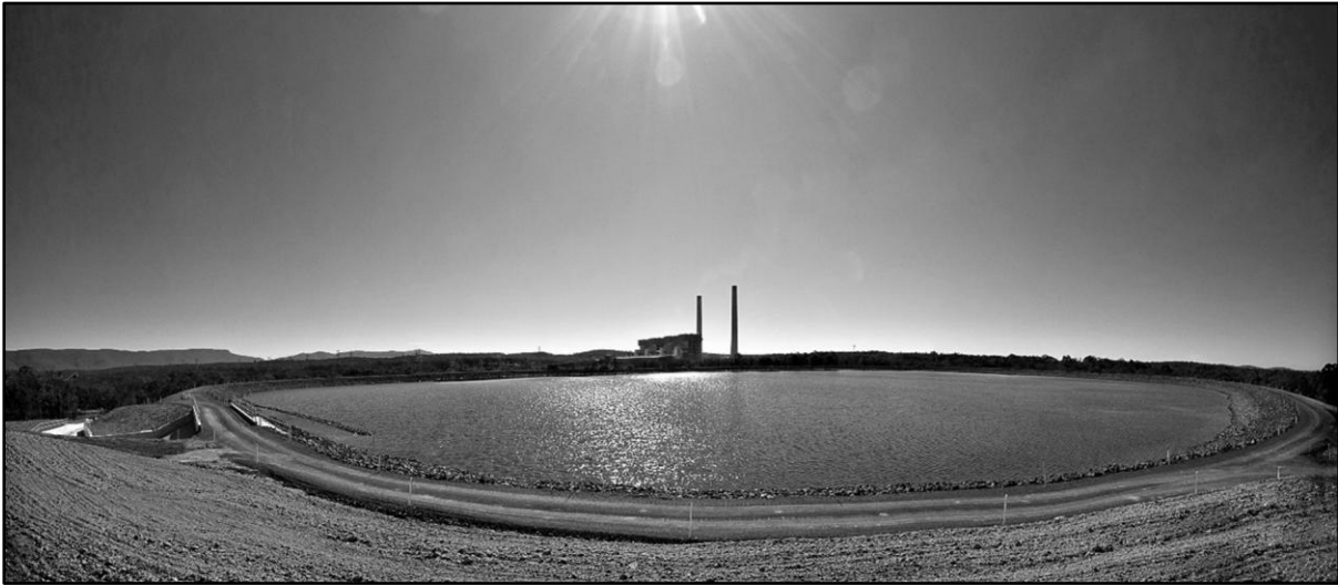
Figure 107 Across the Attemperating Pond (Origin Energy)
