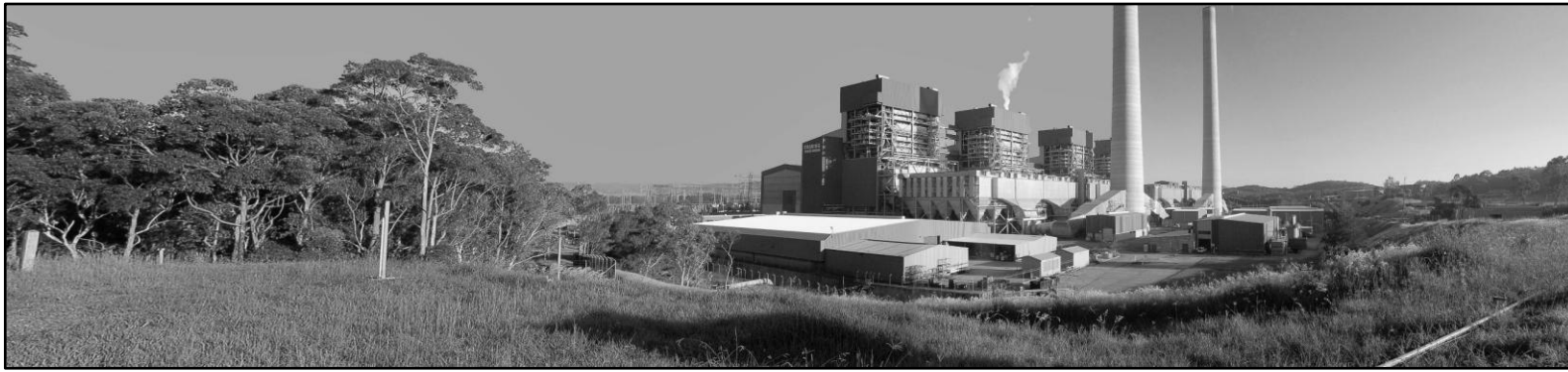
Figure 2 From the south-east, 2007 (Ken Thornton)
