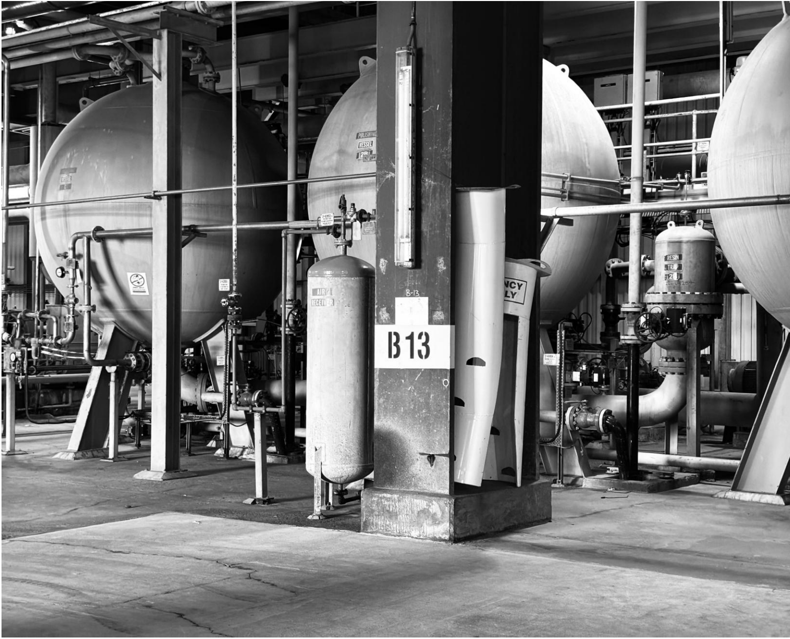
Figure 46 Polishing Plant, January 2025 (Ken Thornton)
