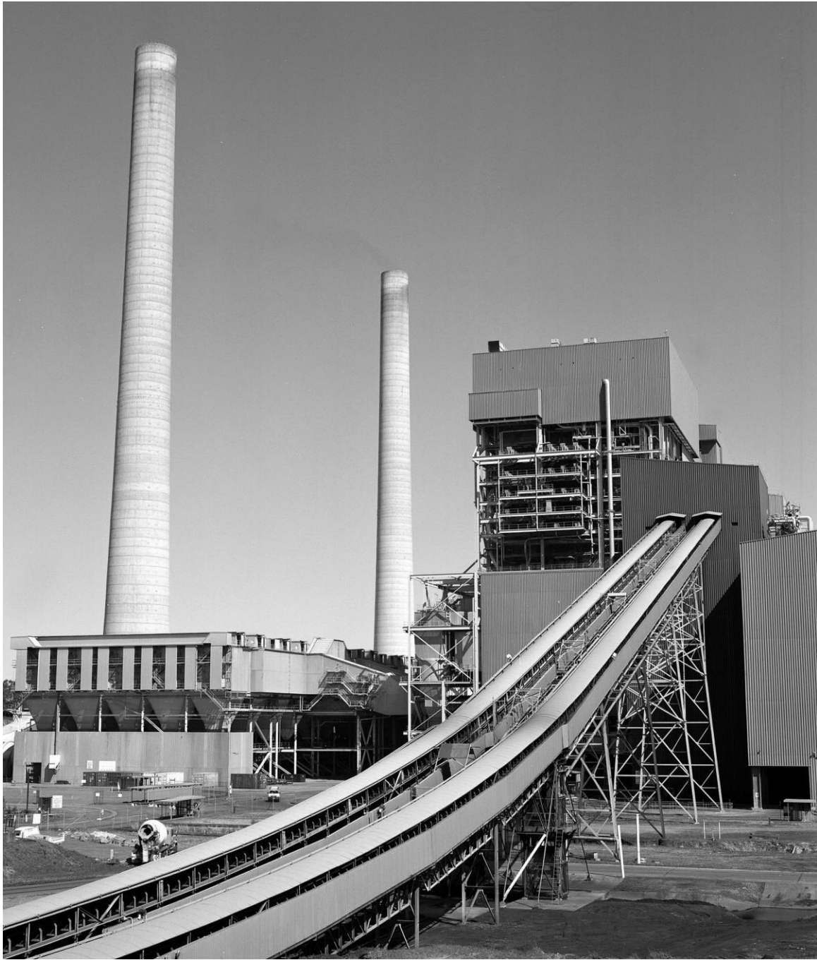
Figure 47 Coal Conveyors (ECNSW)
