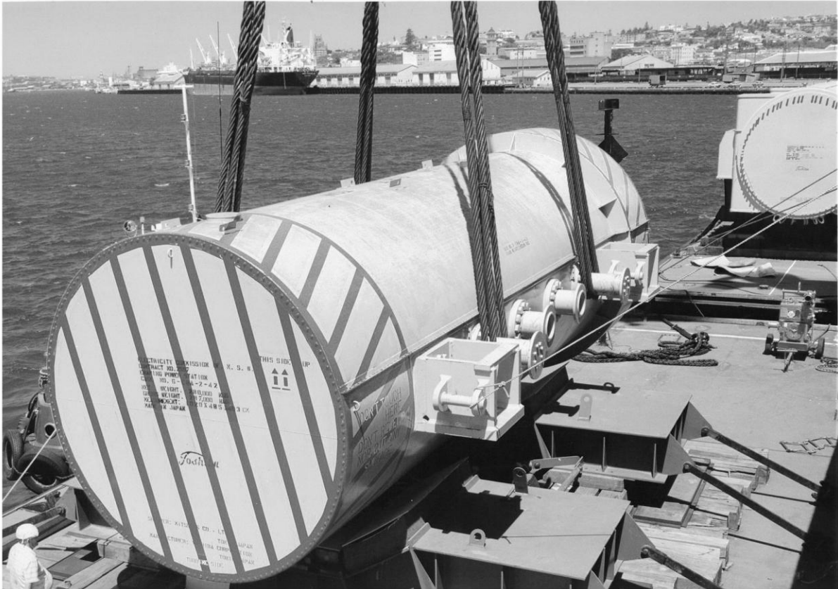
Figure 69 Generator equipment being off-loaded in Newcastle, January 1980 (ECNSW 12357)
