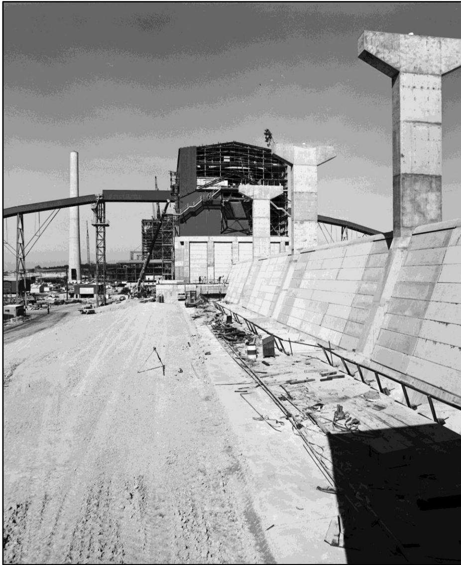
Figure 83 Main Receiving Bin under construction, May 1981 (ECNSW 13406)
