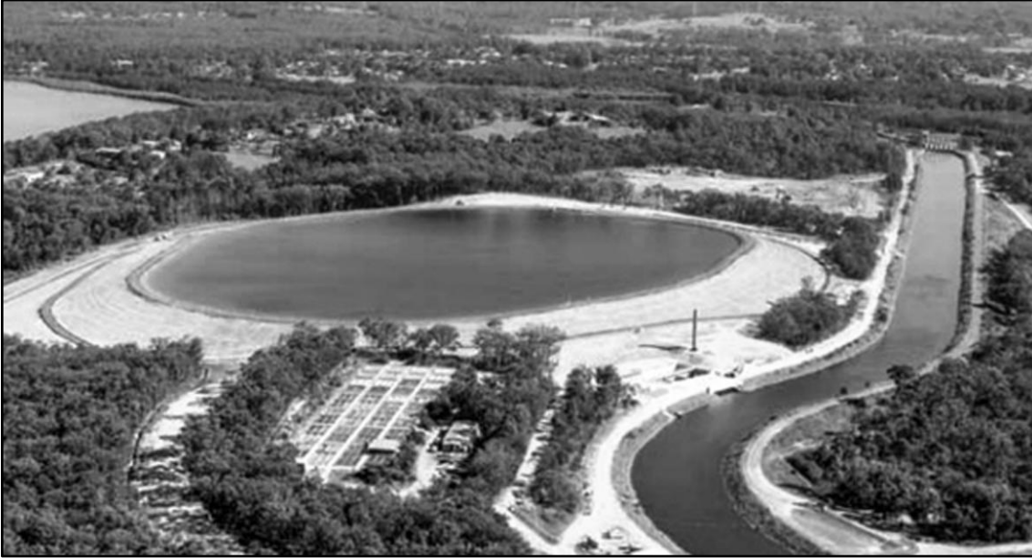
Figure 106 The Attemperating Pond is filled from the High-Level Canal and discharges into it when the outfall canal water needs to be cooled. (Eraring Energy)
