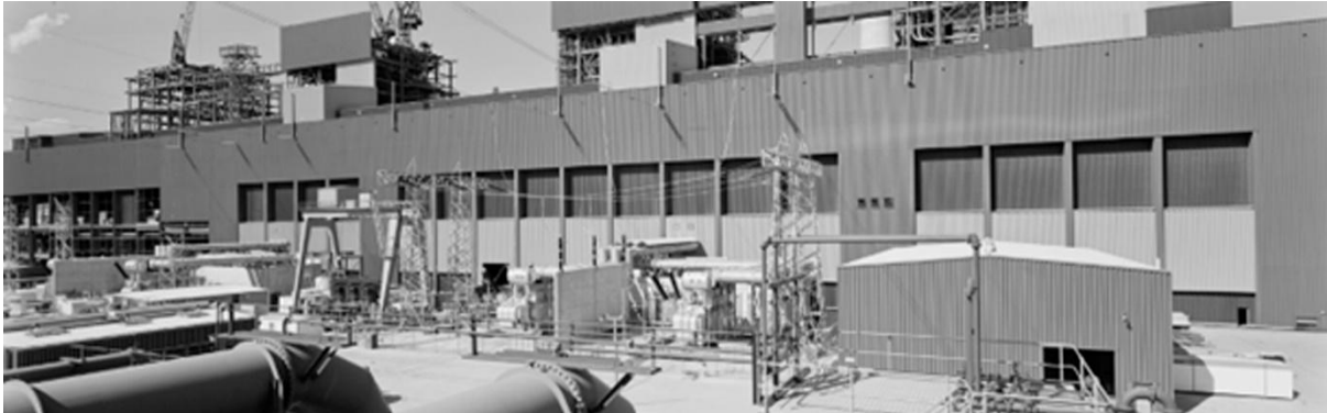
Transformer Bays, March 1982, (ECNSW 13507)
