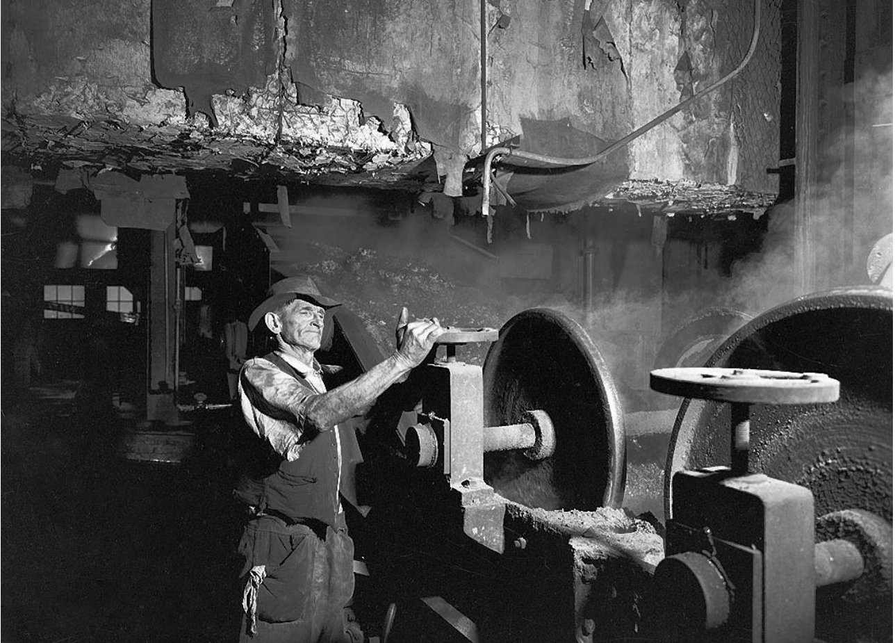
Working conditions were not as they are today, May 1960 (ECNSW 02599)
