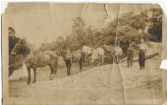
Horse team snigging girders at Mortons Creek
