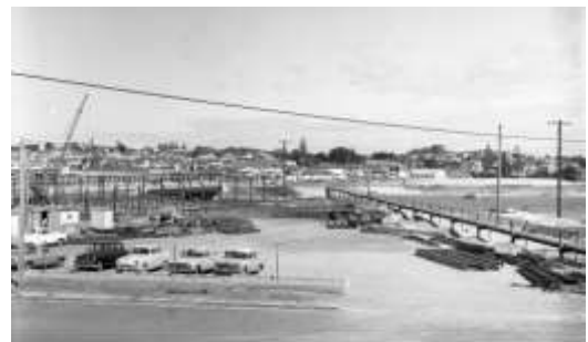
Plaza Shopping Centre Construction
