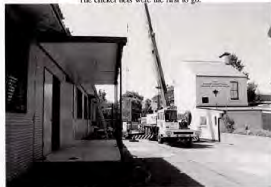
Cranes delivered the demountables.
