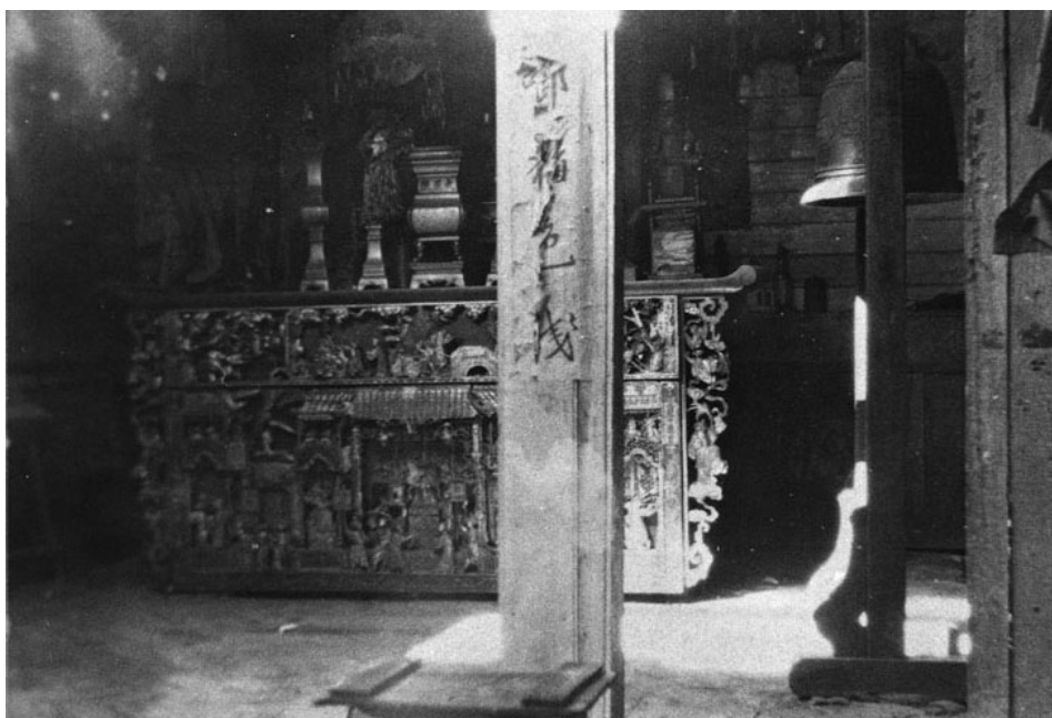
Figure 18. Interior of Rocky River temple, about 1908. (Private collection)
