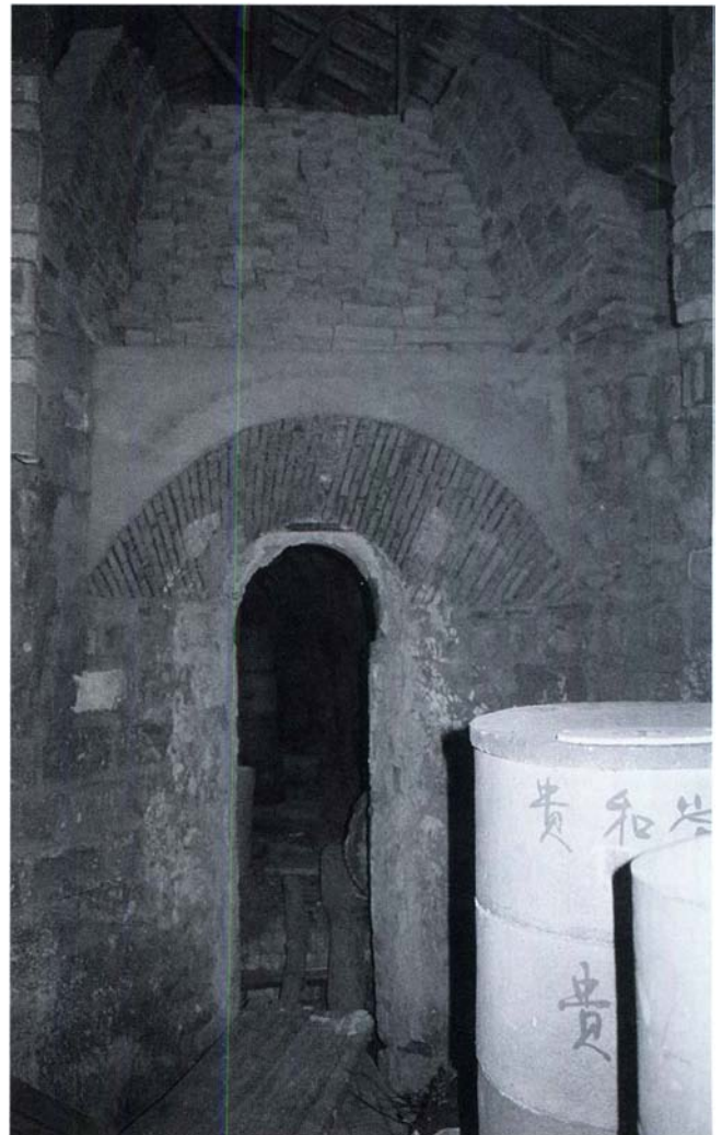
A new wood-burning kiln nearing completion; the arch over the doorway will be left open to serve as a firebox door.
