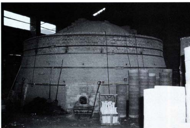
A new downdraft kiln is fired with coal to 1400°C (2552°F); the door is on the side opposite the firebox shown.
