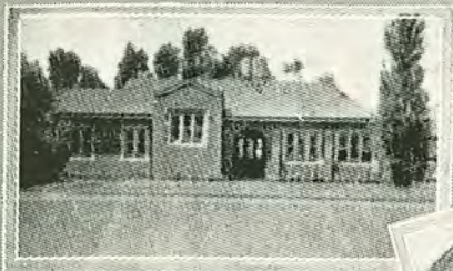
Classrooms Block Northern Aspect
