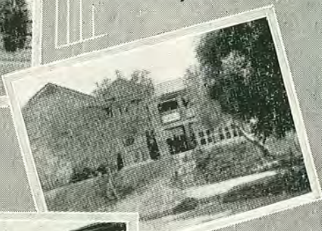
Residential Block overlooking the river
