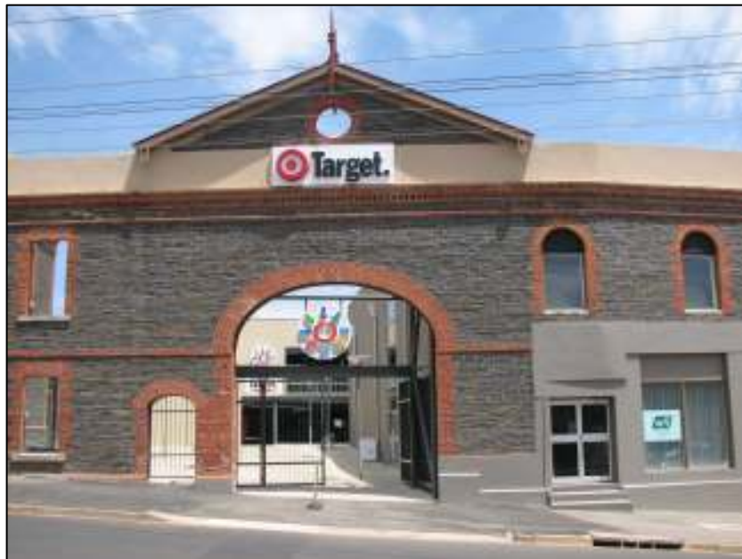
Phoenix Plaza, Calton Road, Gawler East, 2009 (Town of Gawler, Gawler Heritage Collection)
