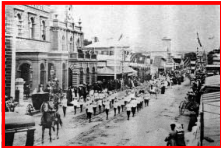
Murray Street, Gawler, 1907 (Town of Gawler, Gawler Heritage Collection)
